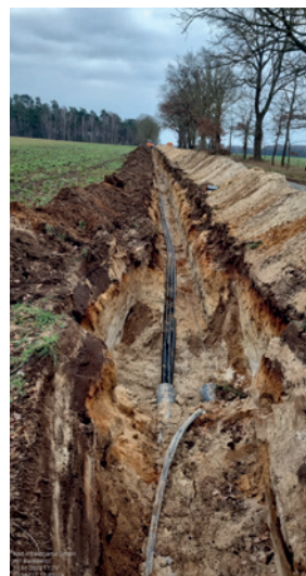
Construction of a cable line in the Bankewitz wind farm
