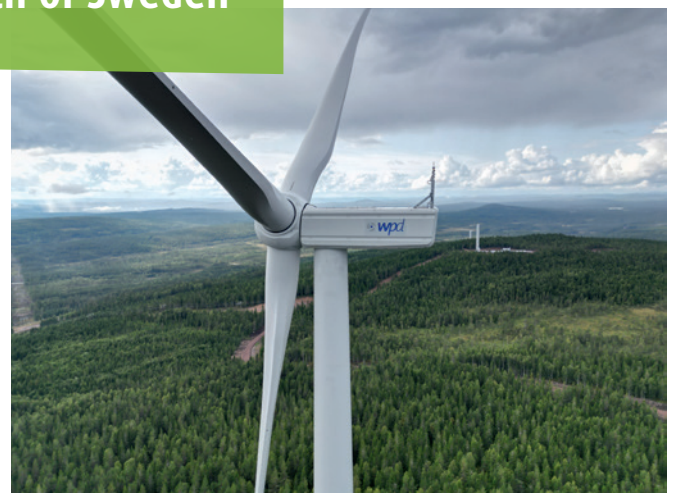
Wind farm Stölsäterberget realized by wpd in 2023
