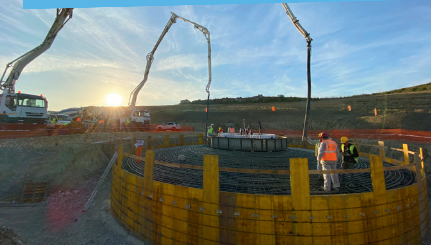
Construction work on Sicily
